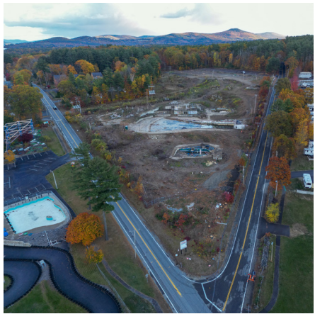
100 ft Grade Change Across the Site
