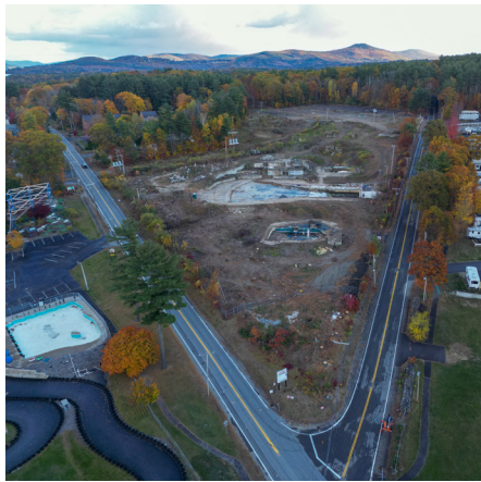
100 ft Grade Change Across the Site
