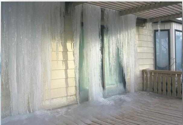
During the cold winter months, broken pipes sometimes occur after the water in them has frozen. Water expands as it freezes, and if the water is trapped inside a pipe with no escape, the expanding ice will cause the pipe to burst. Cracks may appear along the length of a pipe or joints may break away. A burst water pipe can release thousands of gallons of water causing a great deal of damage to your home.
